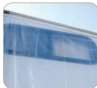
Plastic sheeting protects the sidewalls.
