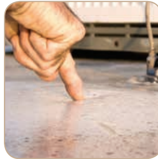
A soft lump in the roof could indicate a concern.
