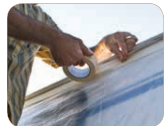
Mask off sidewalls to protect graphics.
